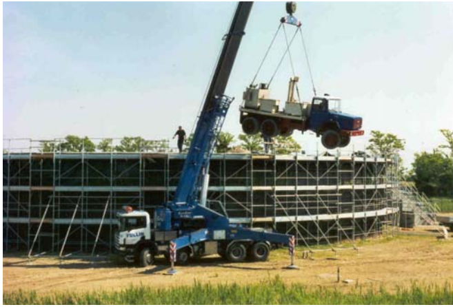
Fig. 9. Positioning of the penetrometer truck for testing after embankment construction
