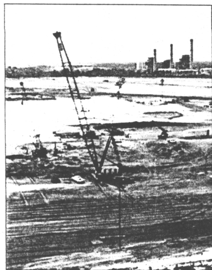
Dynamic Deep Compaction involved dropping heavy weights 100 ft from specially rigged cranes.
