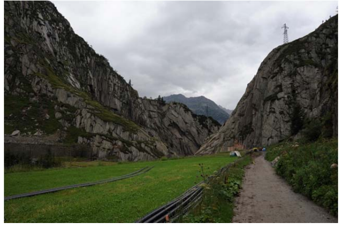
Fig. 5. View over the roof of the avalanche protection gallery with the rock ridges at the gorge to the north.
