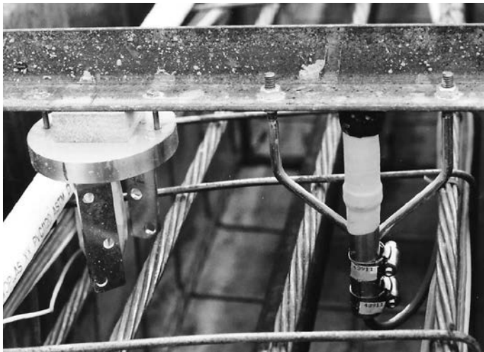
Fig. 3. DMT cell and piezometer in pile form
