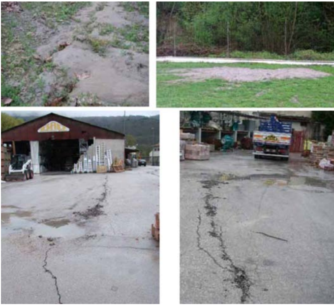
Fig. 1. Evidence of liquefaction (sand boils, ground fractures) observed at Ponte Rasarolo in post-earthquake (April 2009) field reconnaissance (Aydan et al. 2009).
