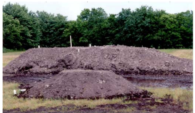
Figure 6: Embankment load test setup
