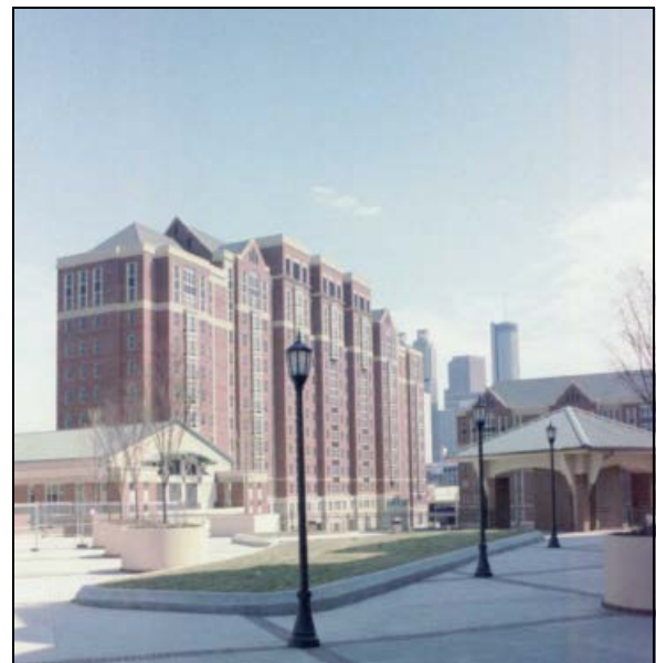
Figure 5. Completed Dormitory Building B
