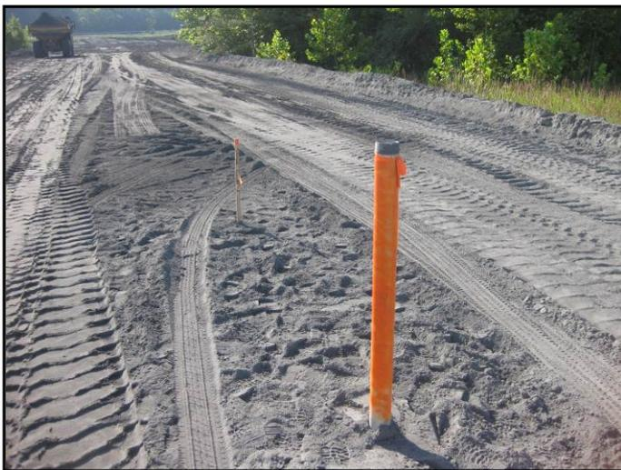
Figure 5B: Completed Settlement Plate--Long term Monitoring
