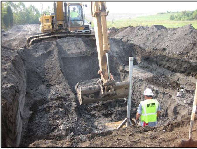
Figure 5A: Settlement Plate Installation
